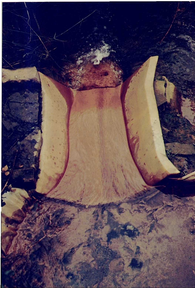
PLATE 1.1 B : Ferric hydroxide deposits on the trapezoidal flume at the Independent Level.
