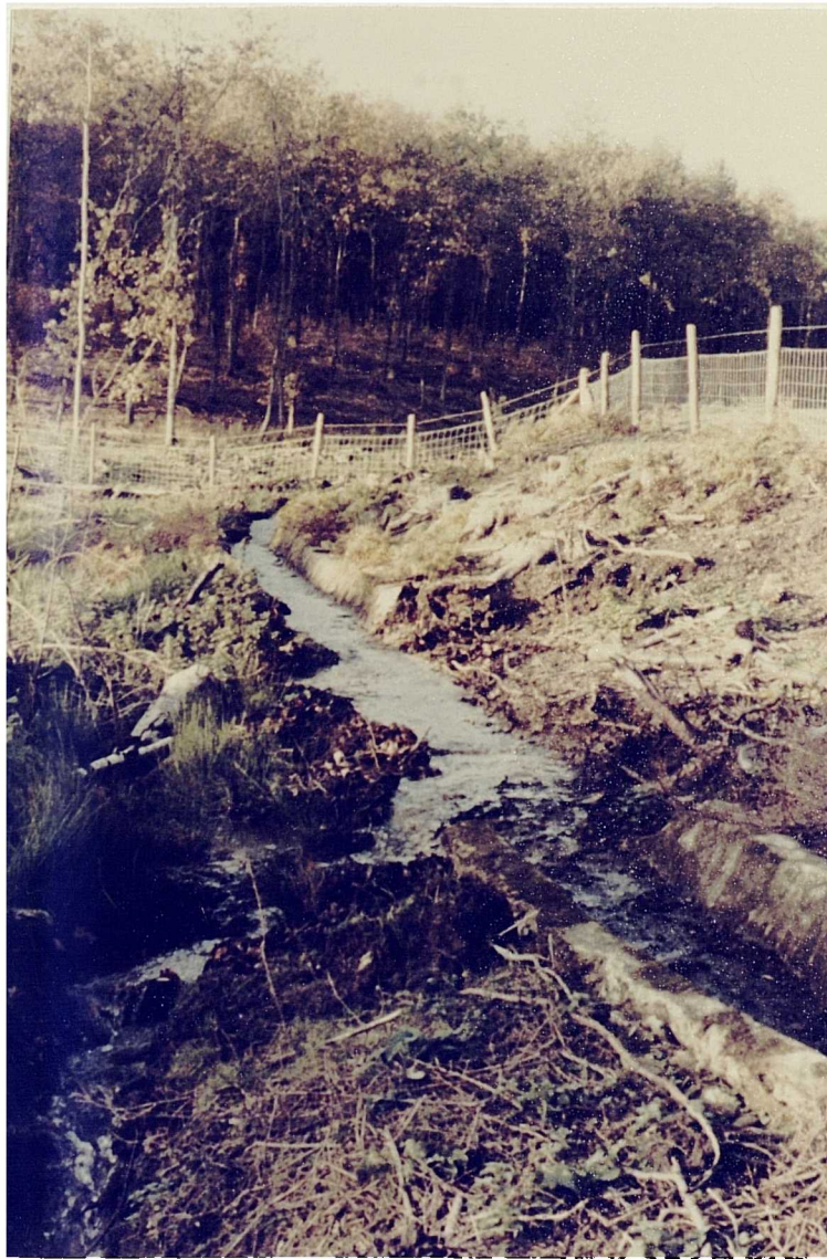
Plate 10.1 : Lined channel of a tributary to the Cannop Brook which flows over the Pennant Sandstone outcrop area. A section of the channel has been destroyed by recent forestry operations and the complete discharge ( 5 \text{ l s}^{-1} ) is completely captured. The discharge is lost by infiltration through the thin arenaceous soil cover over the Pennant Sandstone.
