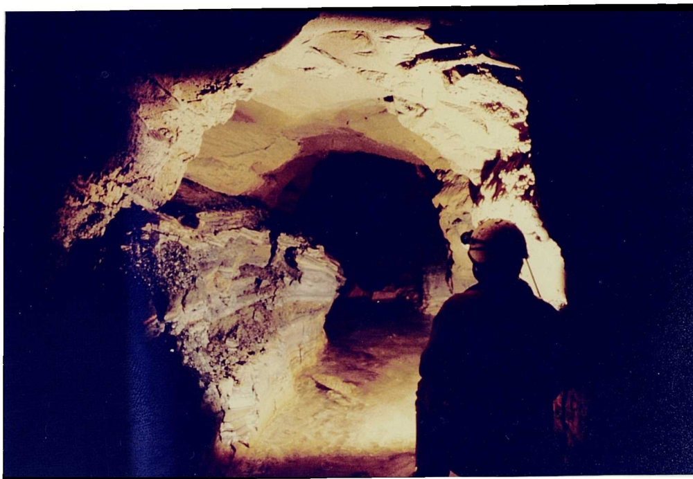
Plate 6.3 : Sediments deposited behind the blockage collapse in the Old Furnace Level.
