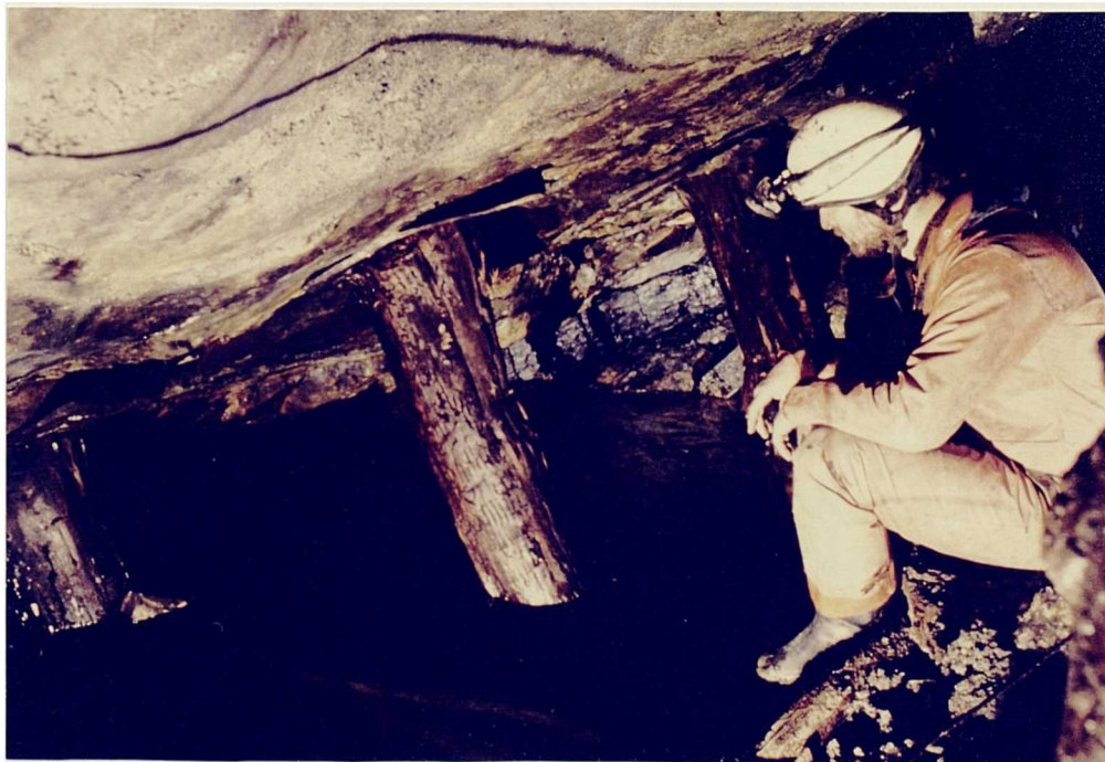
Plate 6.5 : Partial barrier removal | has occurred in the Yorkley coal seam at an elevation below the Old Furnace Level main cross measure driveage, ponding occurs as the intact coal retards further down dip percolation. However, drainage can occur through the overlying fractured Pennant Sandstone into the deep basin.
