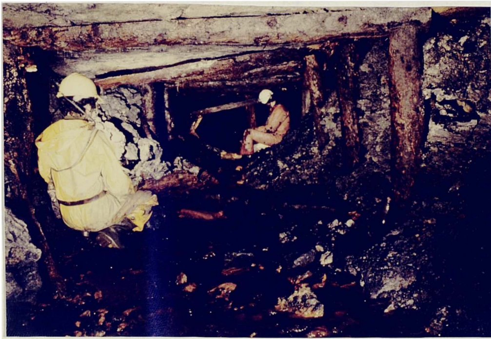
Plate 2.4 : Free-drainage level in coal workings abandoned in 1956 (Miles Level, Forest of Dean). Closure of the adjacent mined void galleries by swelling of the seat earth has occurred, but the competence of the small stream keeps the roadway open.
