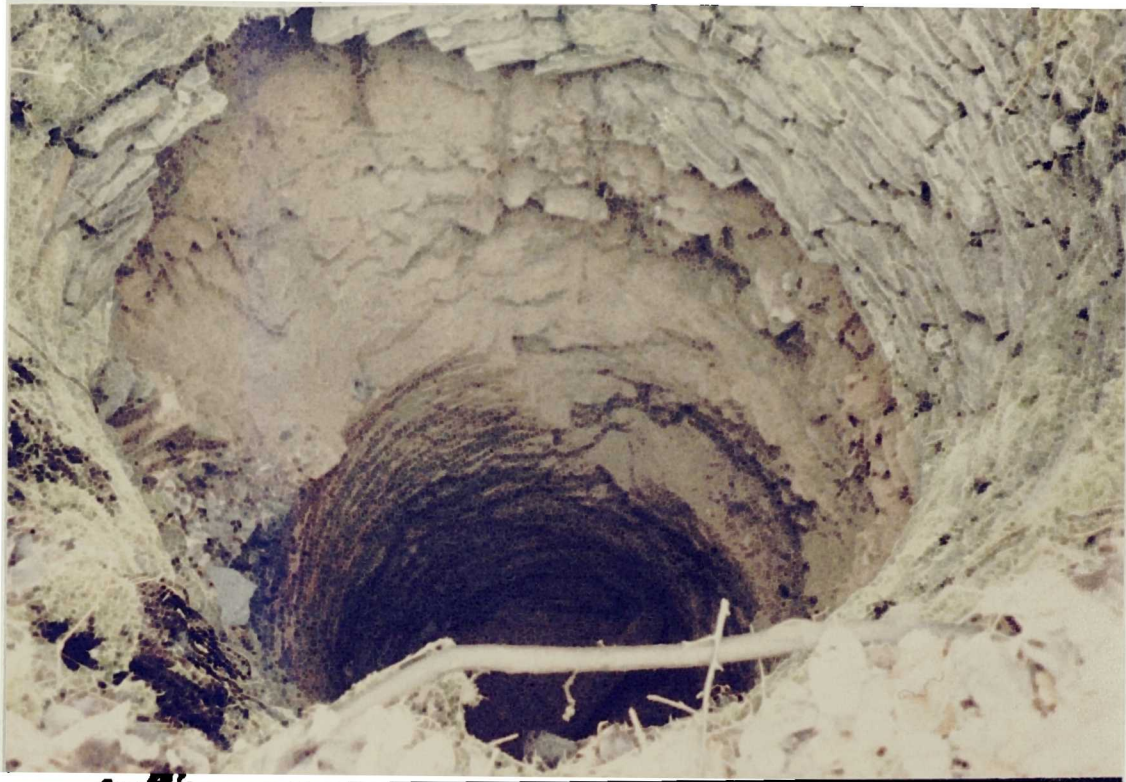
Plate 4.1 : Collapsed shaft in the Miles Level Gale area, showing the accumulated debris cone, a few metres below the surface. The brick lined retaining wall has also collapsed, and the remaining surface masonry appears to be in a precarious state. Numerous shafts such as these exist in the Forest of Dean, but their condition precludes the extensive measurement of rest water levels.
